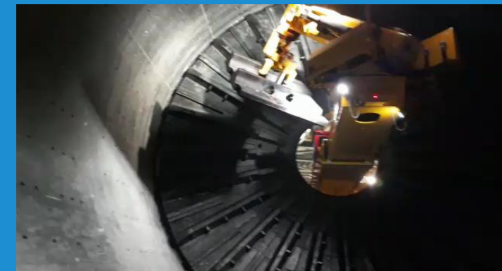
LINER INSTALLATION VIDEO
