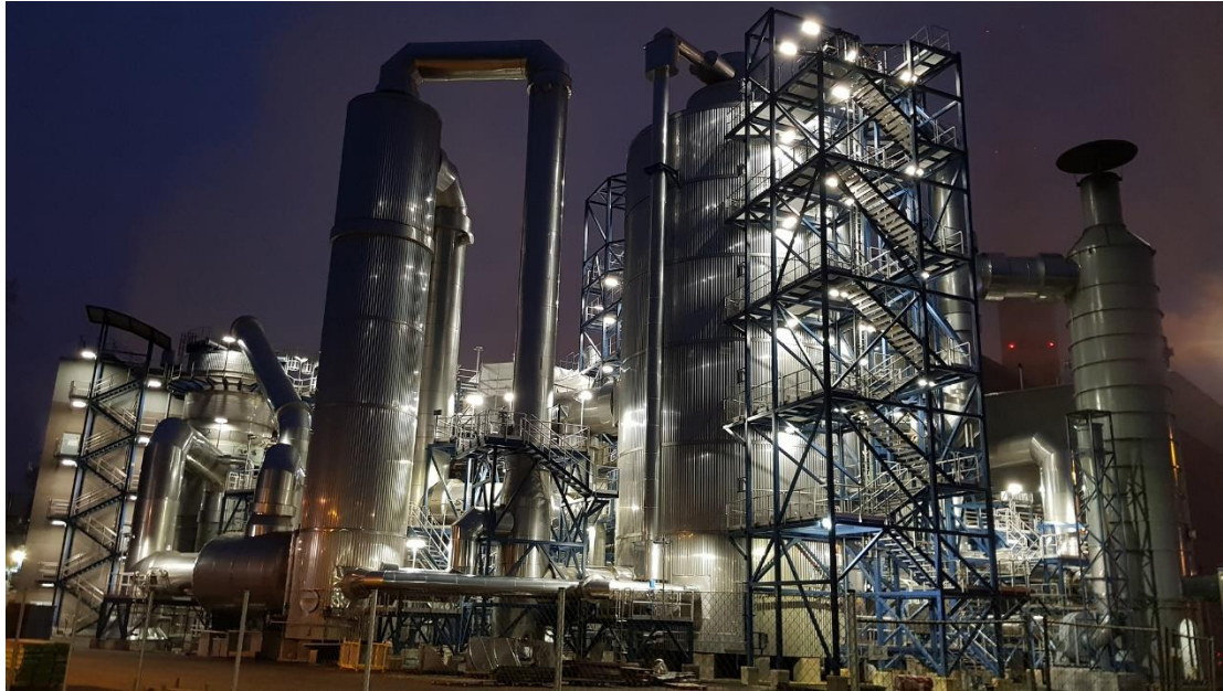
Harjavalta acid plant
