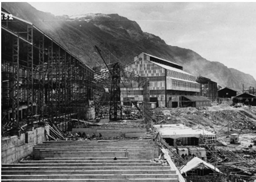
◀ A rapid expansion of the industrial area allowed the establishment of Det Norske Zinkkompaniet in Odda in 1924.
