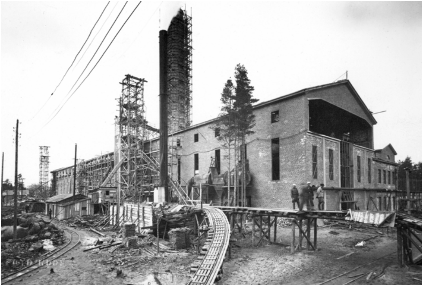
The new smelter in Harjavalta taking shape.
