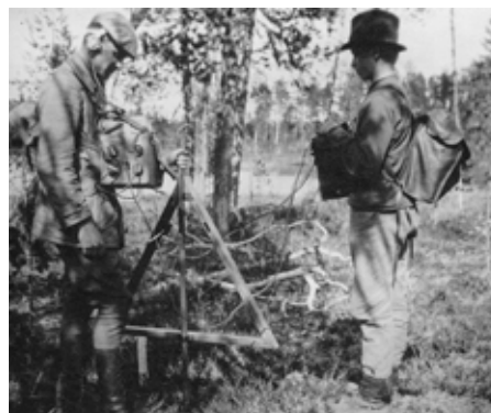
▲▲ Slingram measuring in progress, 1955.
