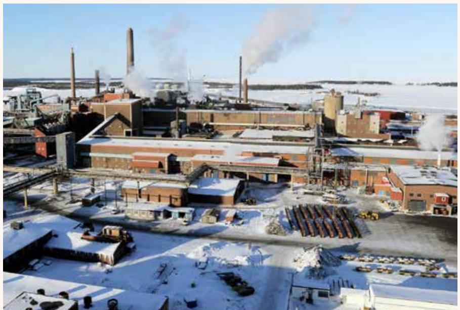
The fire in the electrolysis plant in June, 2023, was Sweden’s biggest ever industrial fire. Right: the area before the fire.
